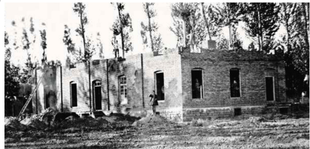
Figure 7. The Westminster Hospital Under Construction (1880–1882) in the Missionary Land Outside Urmia.
