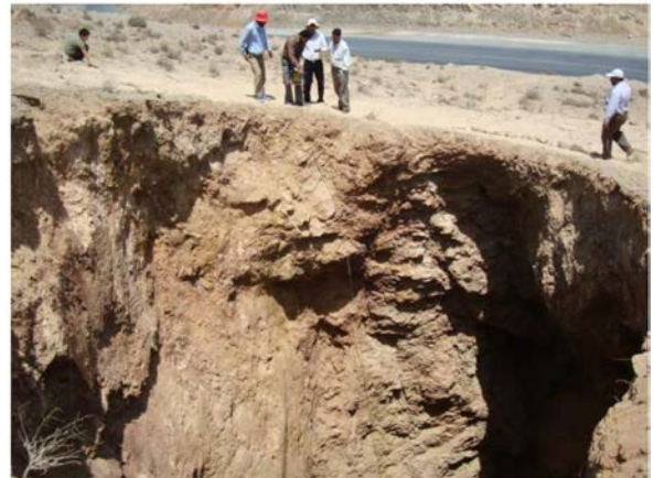
Figure 1. Creating sinkhole in Sormagh (50 m diameter and 16 m depth).
