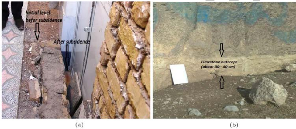
Figure 3. (a) Prolapse in rural houses (20 to 30 cm). (b) The limestone or calcareous outcrops (Hossein mountain's bedrock) on the hillside of Hossein mountain near Shul village (30-40 cm).
