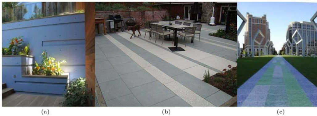
Figure 4. Precast down-cycling: (a) Planters [32]; (b) decks [65]; and (c) pavers [64].
