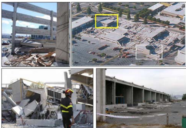
Figure 8. Precast concrete failures in past earthquakes.
