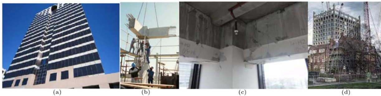
Figure 13. Precast emulative tower [62]: (a) Exterior; (b) construction; (c) typical seismic damage; and (d) demolition.
