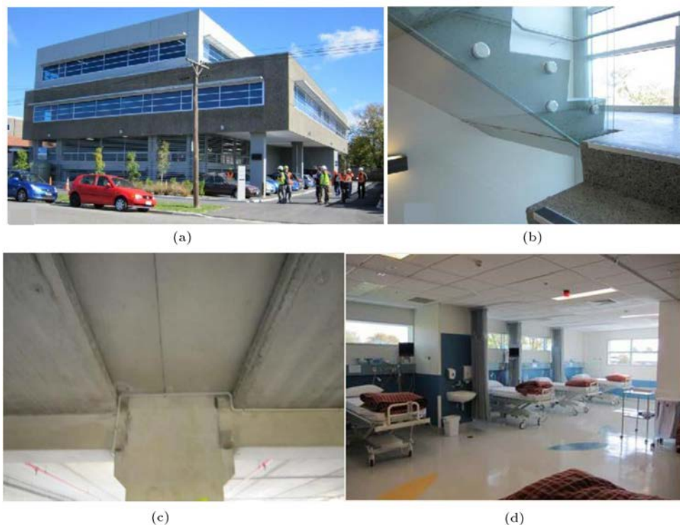
Figure 14. Precast hybrid structure [62]: (a) Exterior; (b) seismic damage; (c) frame; and (d) post-EQ operational.
