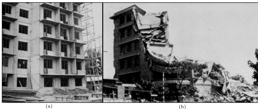
Figure 9. Chinese construction circa 1970: (a) Precast construction; and (b) earthquake damage [52].
