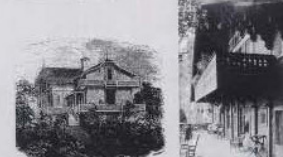
Figure 6.3A. Thomas Clark (c. 1830). A. J. Downing's Architecture/Country House (1845), cited by Matthews in this text. Figure 6.3B. The two-story "Falls" Church designed for the town, November 1833. One of both images courtesy of National Academy of Arts and Culture, Eastern Washington State Historical Society.
