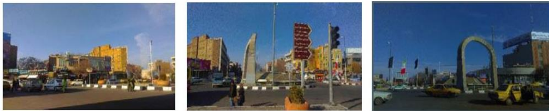
Photo of the current condition of Sa'at square
