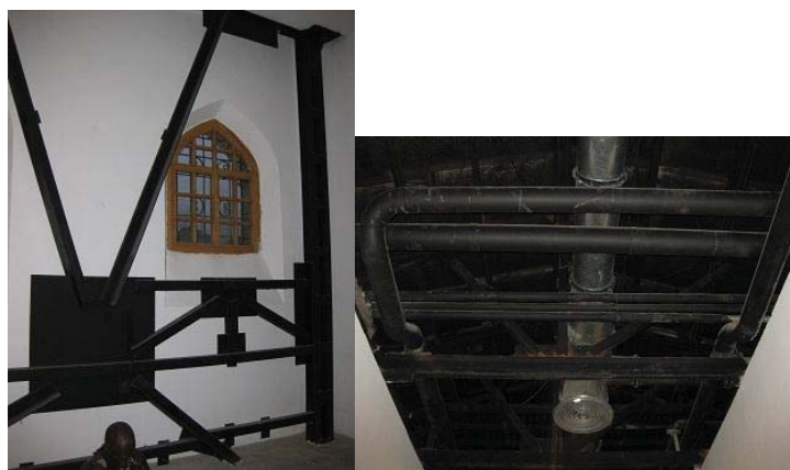
Figs. 48 and 49 Visible attached structure and installations
