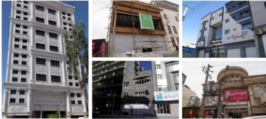
Fig 14. The heterogeneity and turmoil in today's urban construction in Zahedan
