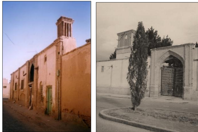
Fig.11 Houses built by Yazidis in Zahedan, with windscreen and brick decorations
