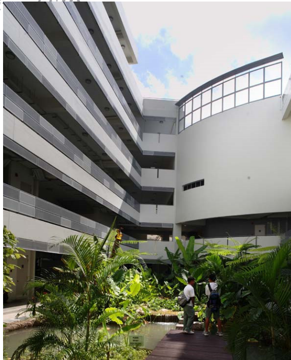
Fig. 7. Close relation between outdoor and green space and educational space in NUS high school in Singapore (Design share, 2018)
