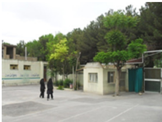
Fig. 13. Poor quality and improper design of outdoor space in Niayesh high school
