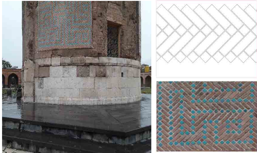
Fig 8. The brick work pattern and execution The construction line in the body of Sheikh Haider's building (Authors, 2019).
