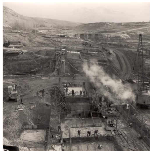
MAHABAD PROJECT No. 0093 Spillway - Bucket 20.10.47 Bottom Outlet Side 18.1.69
