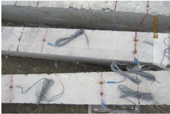
Fig. 11 Strain gauges attached to rubberized concrete
