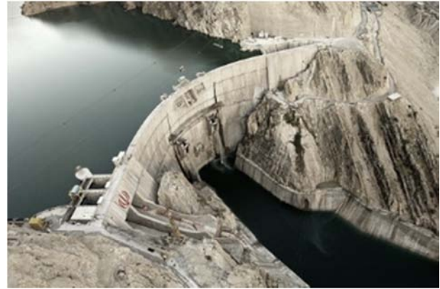
Fig 4 Karun 3 dam and its reservoir and appurtenant
