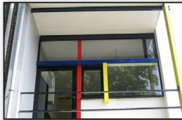
Fig.17. Details of the Schroder House, Architect: Gerrit Rietveld, 1924, in Utrecht, Netherlands. Source: www.greatbuildings.com
