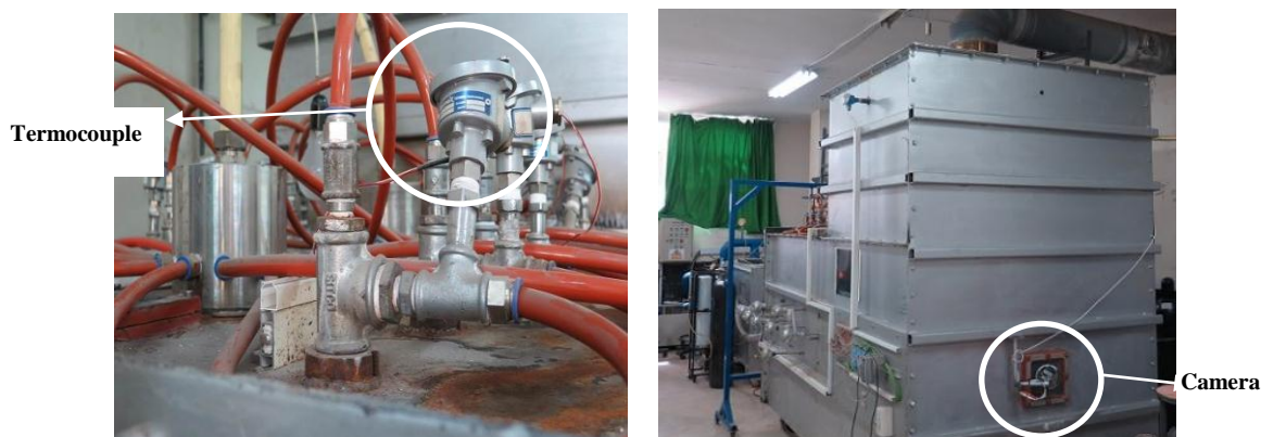
Figure 9- Exhaust Gas Stack and Quench Cooler
