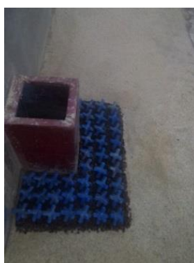
Fig. 6- Placing riprap and SLC on the bed (ARB 1 )
