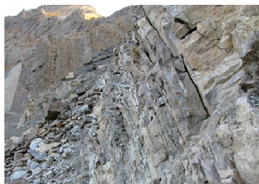
(b) Photo of a failed rock slope
