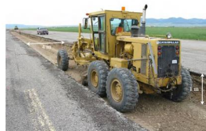
Fig. 1. The filed test trench [23]
