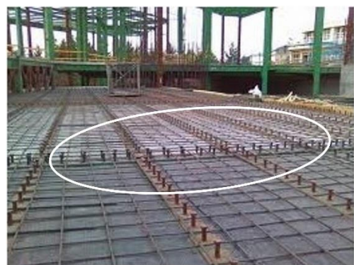
Fig. 1. Composite girder and secondary beams before the construction of concrete slab
