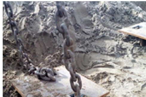
Fig. 2. Attachment of chain to piles for removing them
