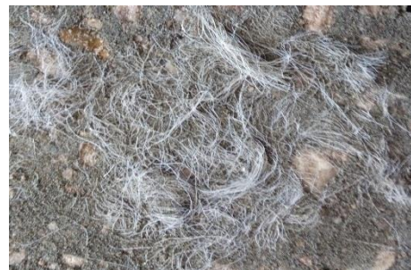
Fig. 6. Flattening of fiber at concrete surface
