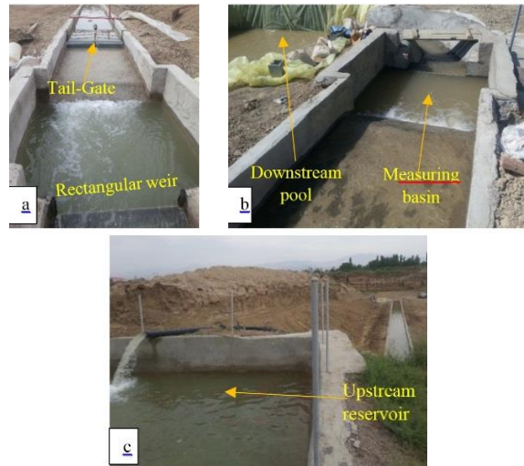
Fig. 3. (a) Rectangular weir and tailgate (b) measuring pond and downstream pool (c) upstream pond
