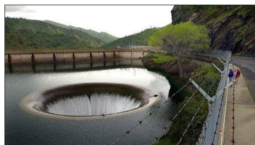
Fig. 1. Sample of morning glory spillway
