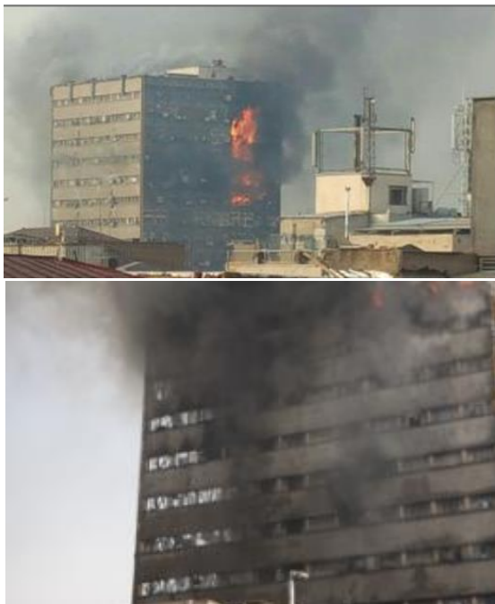
Fig. 2. top: fire development in 10 th to 14 th floors of the northwest; down: northwest building collapse
