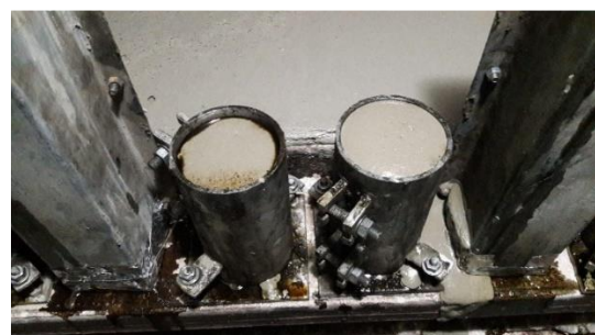
Fig. 2. Sample images in the preheating hall
