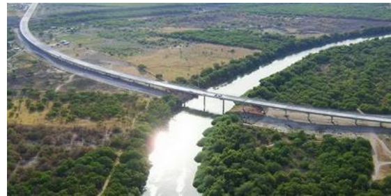
Fig. 1. Rio Grande Bridge, Mexico
