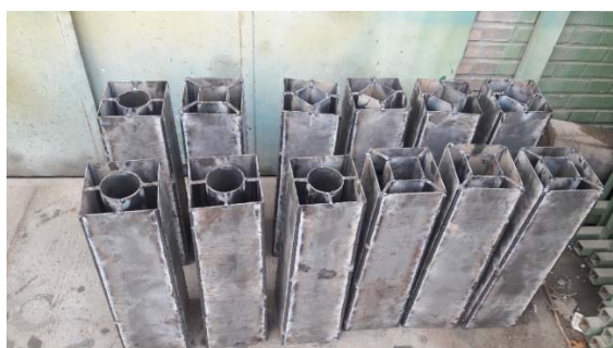
Fig. 2. Columns made before concreting
