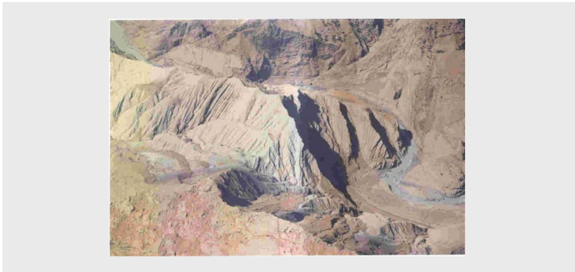
Figure 15- Sample of channel erosion on the entrance of Dez reservoir
