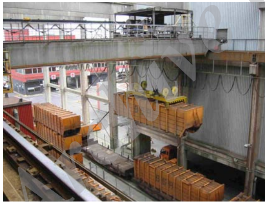
Fig. 3-3.3: Rail Transfer Station in Berlin-Gradestrasse Built by BC-Berlin
