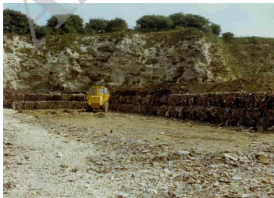
Fig 3-2.3: Land Filling of Bales
