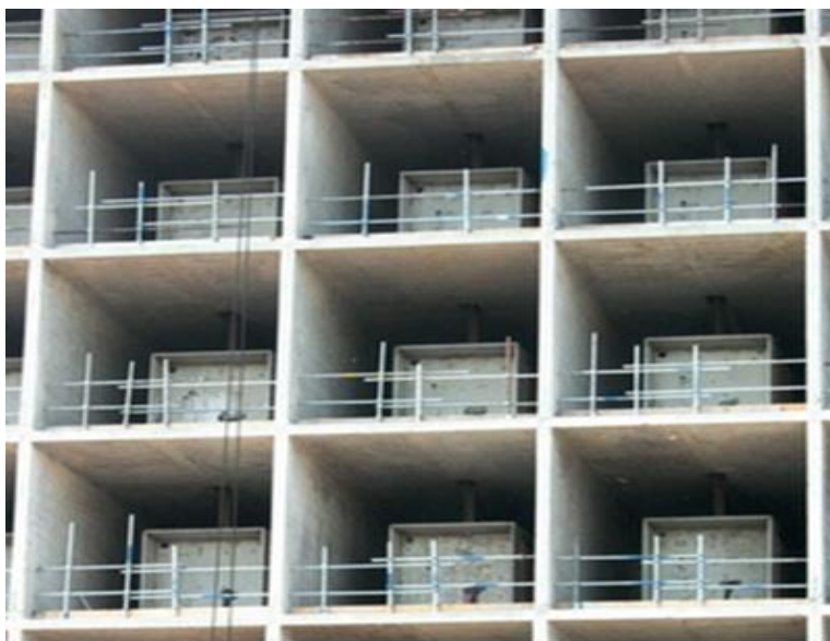
Figure 1. RC wall system
