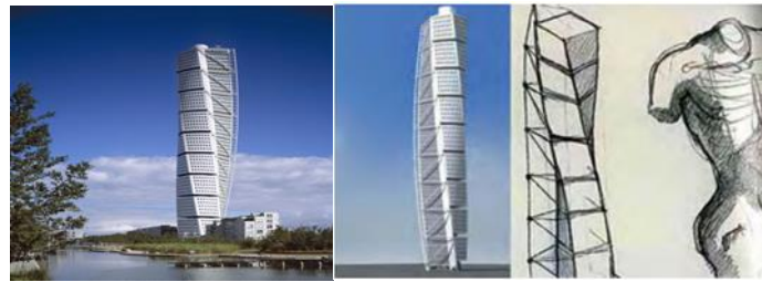
Figure 4. The turning torso residential tower
