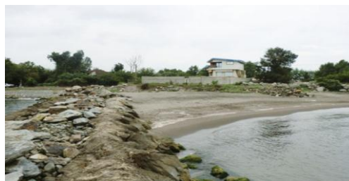
Fig 5. Beach deformation in the vicinity of groyne at Guilan Beach (Afsoos Biria et al, 2014).
