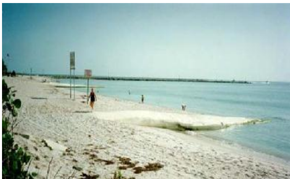
Fig2. Sand-filled Groins Stabilizing a Florida Beach (Harris, 2003).
