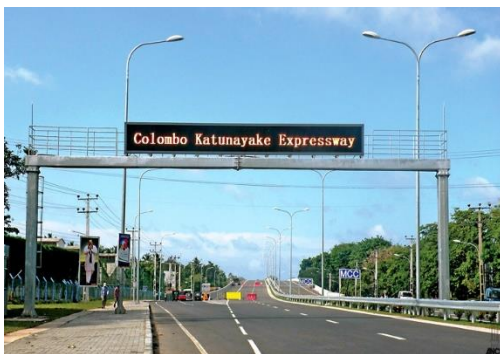
Figure 1- A single row matrix LED sign on Katunayake Expressway in Colombo, Sri Lanka
