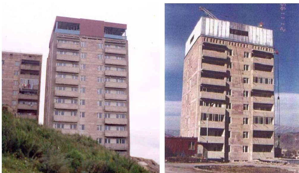
Figure 5- Seismic Upgraded Buildings using AIUF
