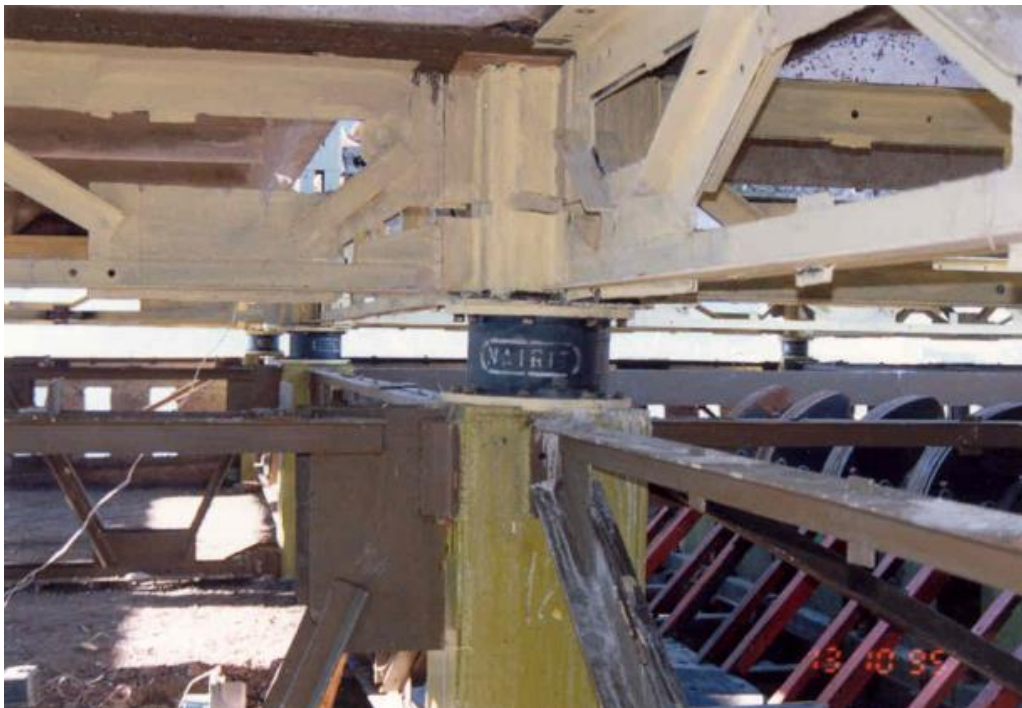
Figure 6- AIUF Implimentation Technique on Roof Floor of 111 Serie building
