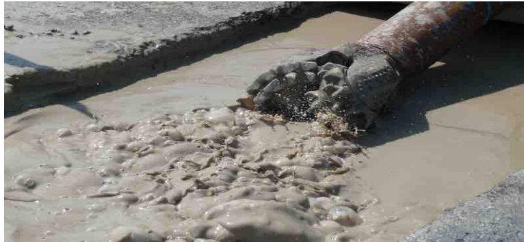
Figure 3: Drilling mud while pulling drill out
