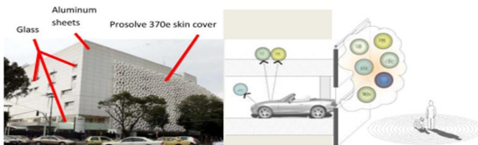
Figure (7) Manuel Gea Gonzalez Hospital using conventional TiO 2 (Prosolve370e — beautiful decorations, decorative facades that "eat" pollution - "incredible smog-eating building" - CNN).
