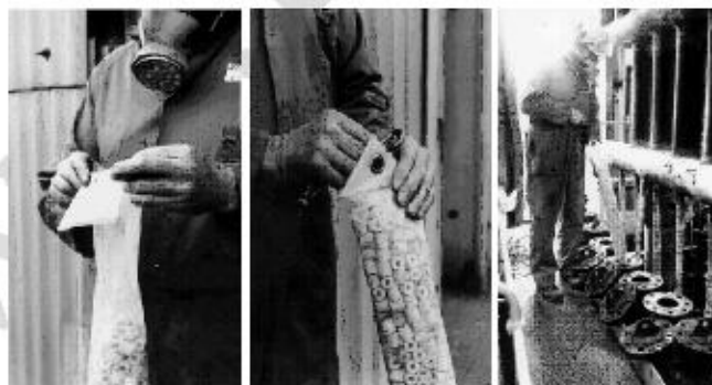
1-folding over 2- attaching rope 3- filling tubes
