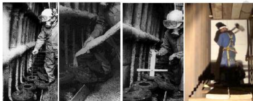
4- jerking rope 5-topping up 6- checking outage 7- hammering for adjustment level
